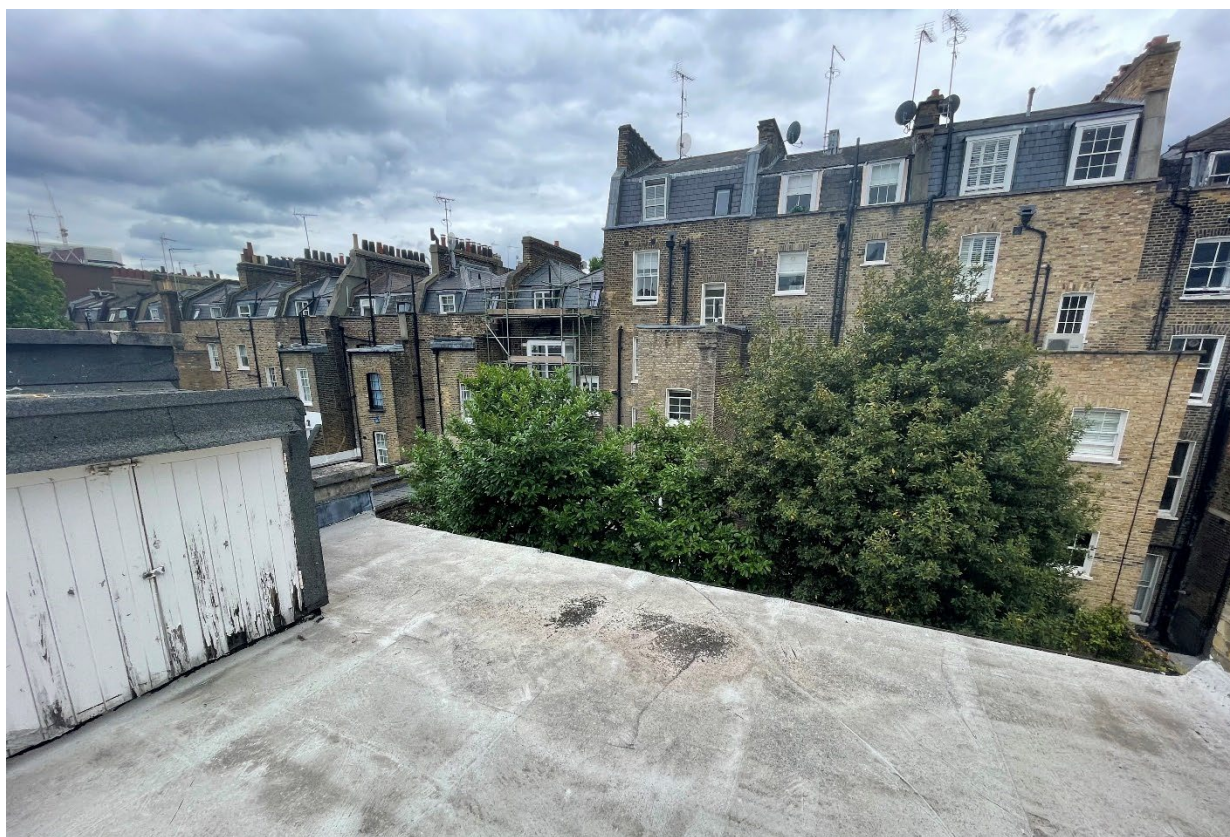
Views from main roof level
