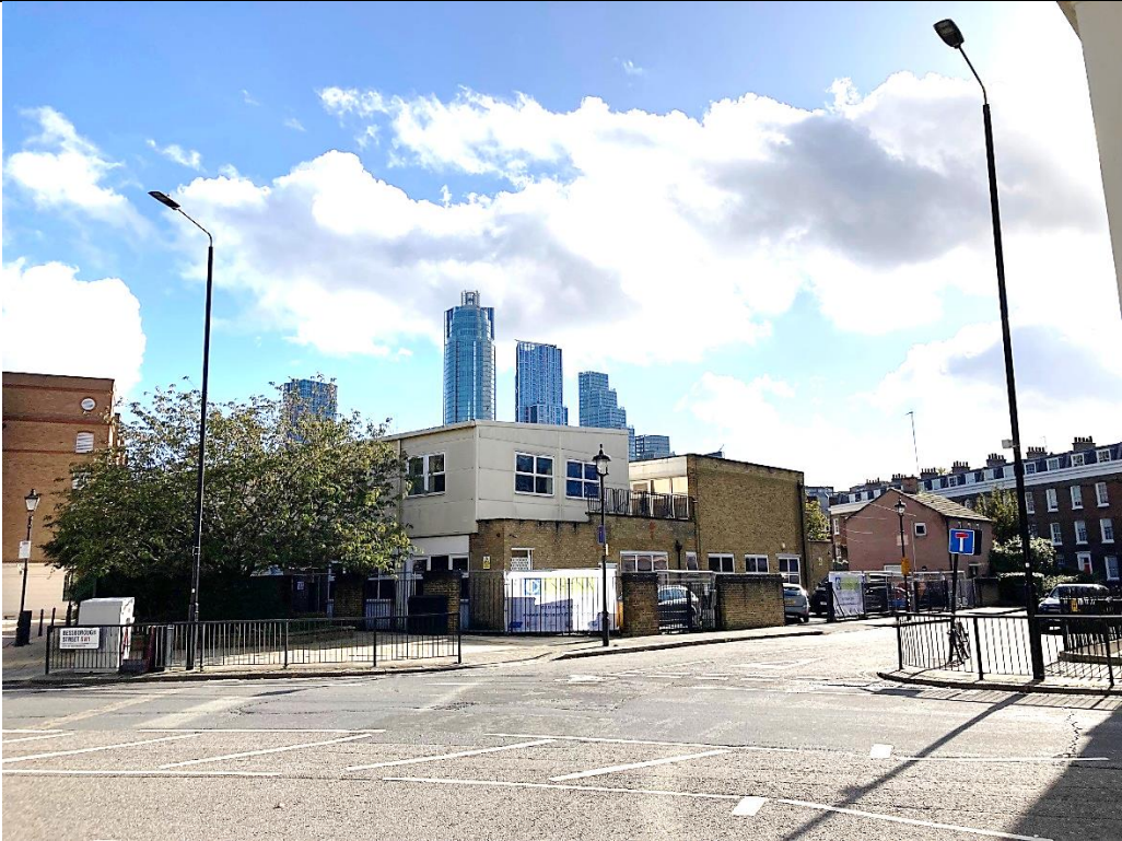
View from Bessborough Street
